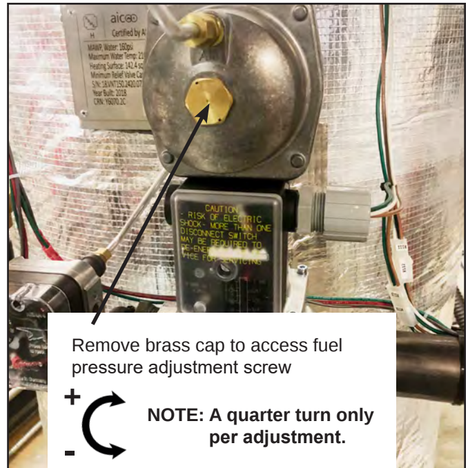
Figure 43. Fuel Pressure Adjustment Screw
