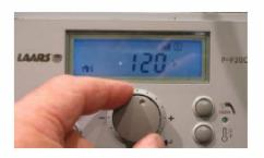
Use the Scroll/Select button and adjust to desired set point.
