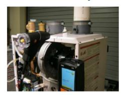
**1.** Connect a manometer to the manifold pressure port. For dual port manometers, use the positive pressure side. Check for proper manifold gas pressure. Refer to Table.
