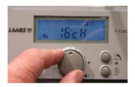
Using the Scroll/Select button locate 16:cH
