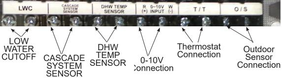
Install and connect the Outdoor Sensor to terminals marked O/S. Then you will need to go to the Installer Parameters to complete the set up
