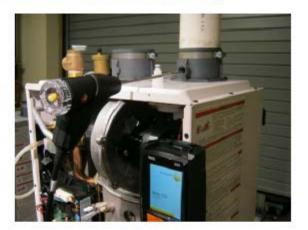
CO2 adjustments are made when the boiler is in "Min Fire"
