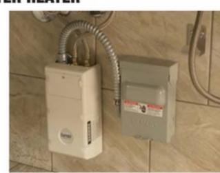
factory-set at 120° F (3.5 kW and below set at 105° F). Special settings of higher or lower range available based on options. Other features include: active energy management with power modulating controls; microprocessor temperature control with digital display for thermostatic accuracy; and flow meter activates heater only on demand.
