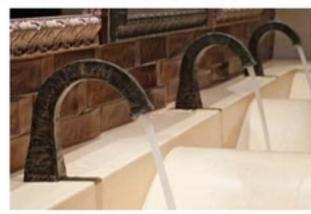
interrupts the electromagnetic field, the faucet valve opens automatically to begin the flow of water.
