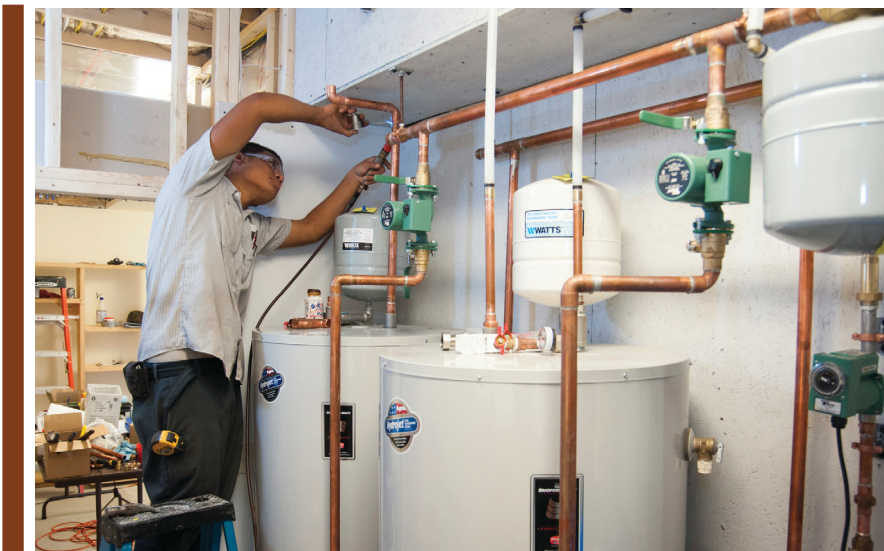
120-gallon Bradford White tanks and Taco circulators
