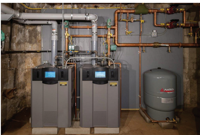
Below. Redundancy, efficiency, and much-improved indoor air quality resulted from installation of the two NeoTherm condensing boilers.
