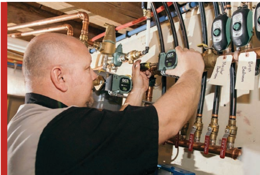
Doug Zerbe, technical manager, replaces the cover on a new Taco 007 circulator during final inspections, and system commissioning.
