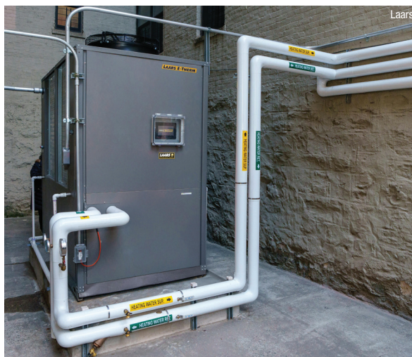
The Laars E-Therm Heat Pump Water Heater installed at 850 Bryant Avenue.
