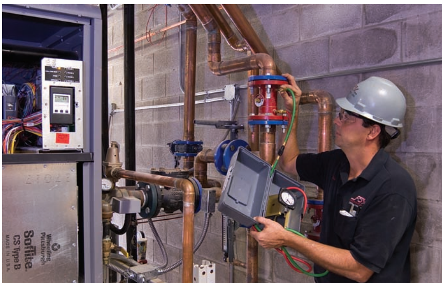
Bill Bosaw, Fox Mechanical field superintendent, is taking a differential reading across a balance valve. This reading indicates the volume of water going to the boiler.
