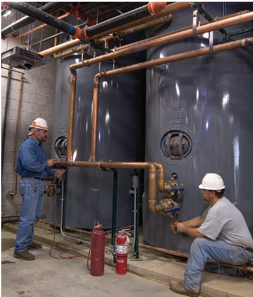
Larry Fast (left), journeyman, and Jim Buyko, foreman, Aggressive Mechanical, complete connections to both of the 2,020-gallon Laars storage tanks.
