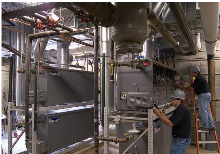
Bill Bosaw, field superintendent, Fox Mechanical, (left), performs a combustion air reading of one of the Pennant systems, while another Fox employee inspects one of the boiler's pull-out control panels during startup, confirming that the control sequence is working properly.
