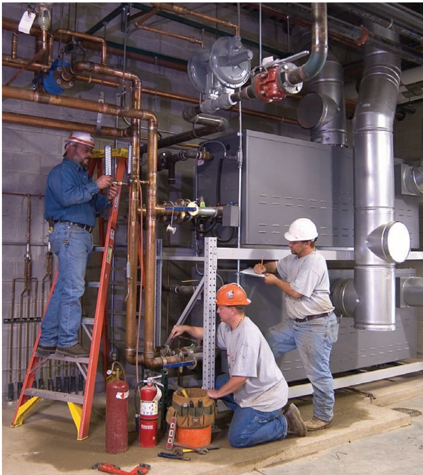
Aggressive Mechanical Journeyman Larry Fast (left), Todd Holcomb, journeyman, and Jim Buyko, foreman, complete the installation of two, stacked boilers.
