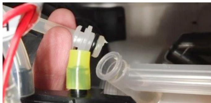
Step 16. Disassemble and clean any debris or build-up from the condensate trap. Ensure the check ball moves freely up and down inside the trap and the clear tube between the condensate trap and air pressure switch is clean and dry. Reassemble and re-install the trap once it is clean and the boiler heat exchanger has been flushed.
