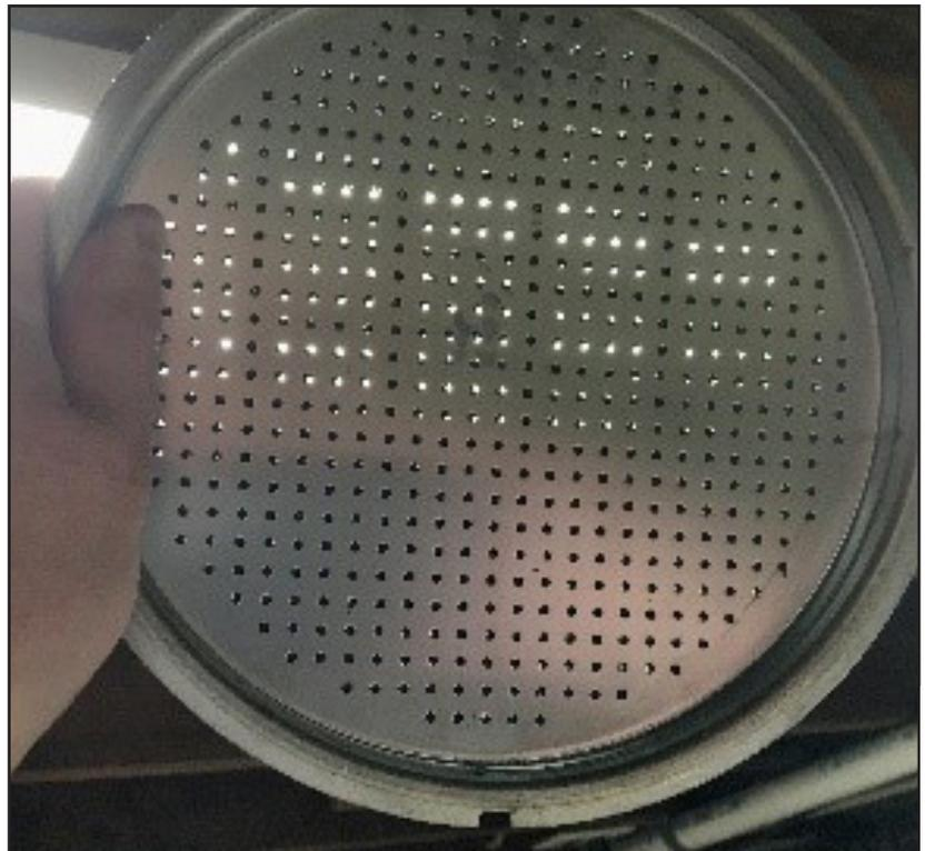
Step 14. Inspect the combustion chamber for deposits and debris. Remove deposits in the combustion chamber with a damp rag – DO NOT use metallic brushes or any type of detergent inside the heat exchanger. Be sure to clean the inside surfaces of the combustion chamber observation window and the flame sensor window.
