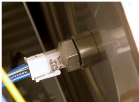
Fig. B21-1 - Stack temperature limit switch (typical)
