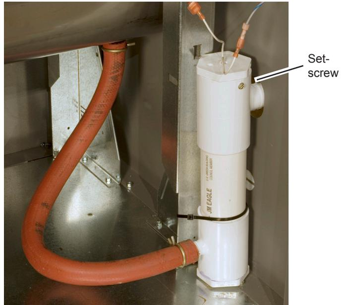
Fig. B13-1 - Small condensate trap assembly (typical)
