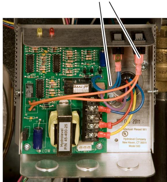
Fig. B6-4 - Control for low water cutoff with cover removed
