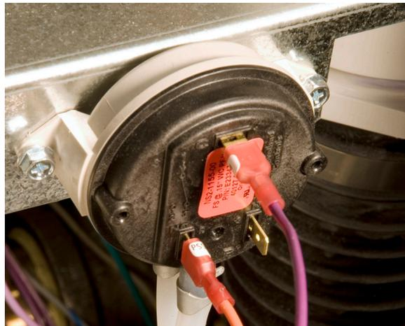
Fig. B17-1 - Air pressure switch (typical)
