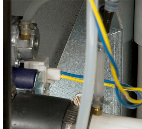
Fig. B11-3 - Wiring connector for gas valve
