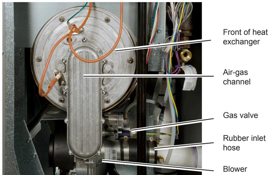
Fig. C5-1 - Front of heat exchanger and other parts (typical - NT105 shown)
