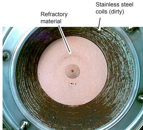
Fig. C5-12 - Dirty heat exchanger
