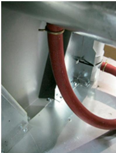
Fig. C5-14 - Drain hose connected under the heat exchanger
