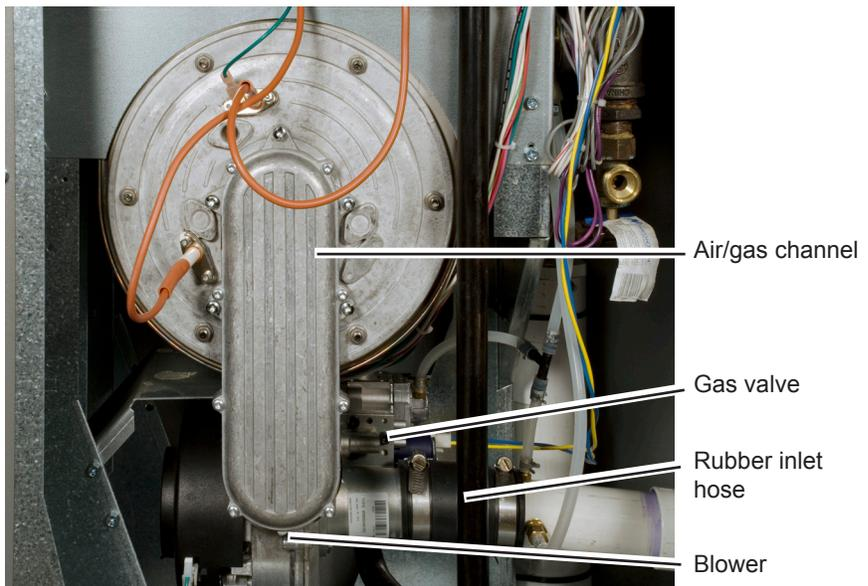
Fig. B11-1 - Gas valve and other parts - NT105 shown
