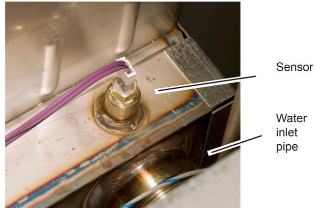
Fig. B24-1 - Inlet water temperature sensor (typical)
