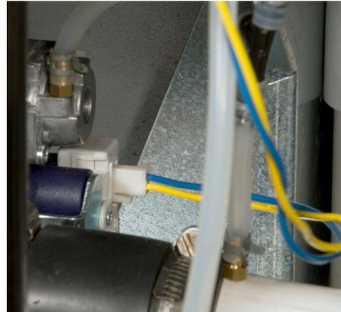
Fig. B19-3 - Wiring connector for gas valve
