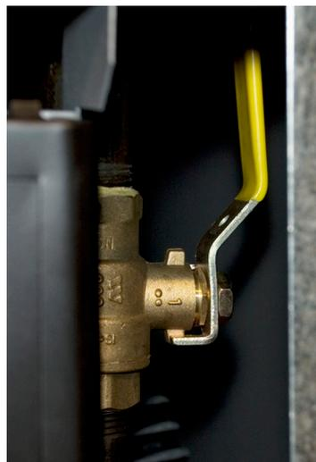
Fig. B11-2 - Gas shutoff valve (typical)
