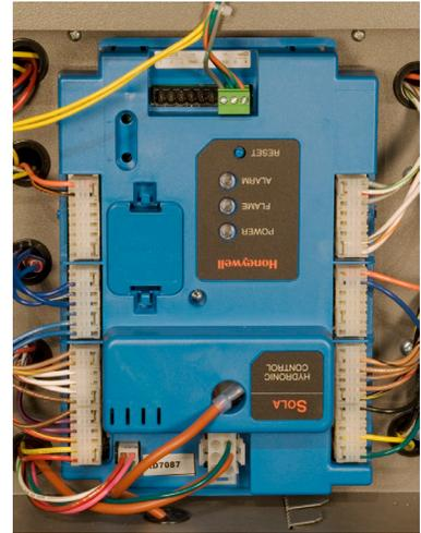
Fig. D9-1 - Honeywell SOLA controller
