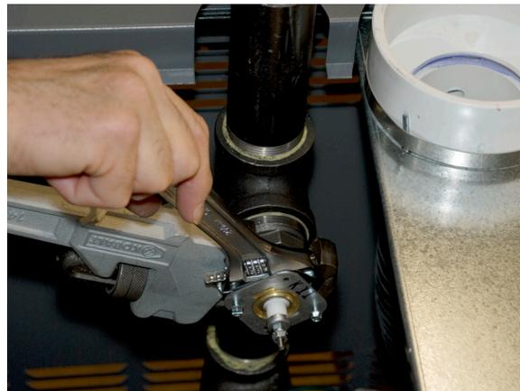
Fig. B6-2 - Removing the probe
