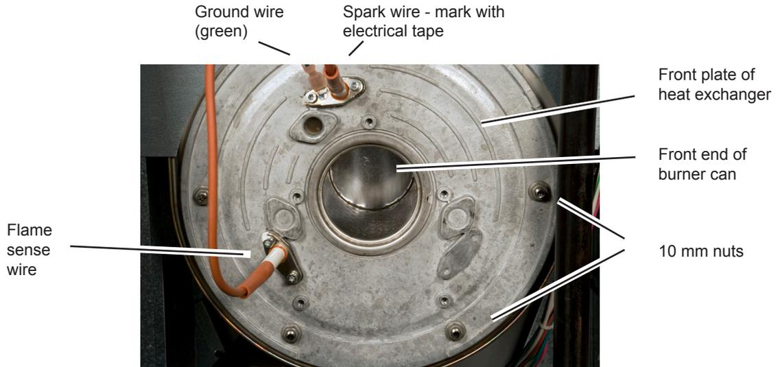
Fig. C5-8 - Front plate of heat exchanger with air-gas channel removed
