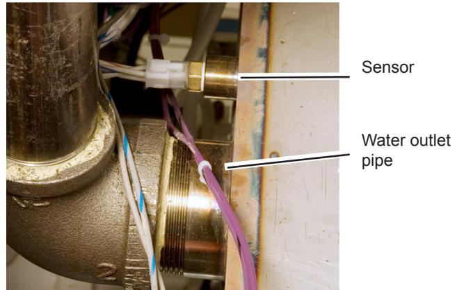
Fig. B26-1 - Outlet water temperature sensor (typical)
