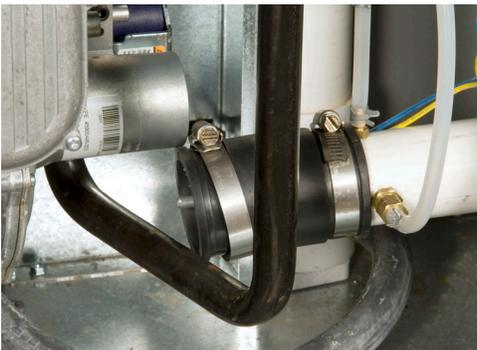
Fig. B19-5 - Loosen the left end of the rubber hose
