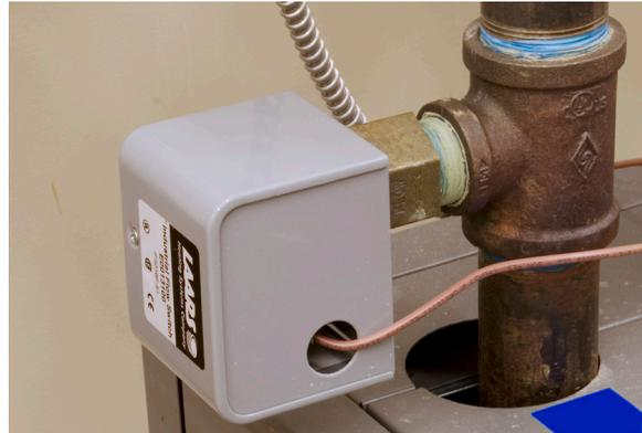
Fig. B10-1 - Flow switch installation (typical)
