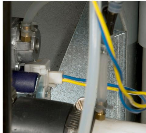
*Fig. C5-3 - Wiring connector for gas valve*
