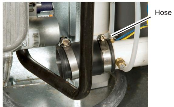
*Fig. C5-5 - Loosen the left end of the rubber hose*
