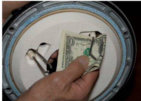
Fig. C5-10 - Correct way to clean the flame sensor
