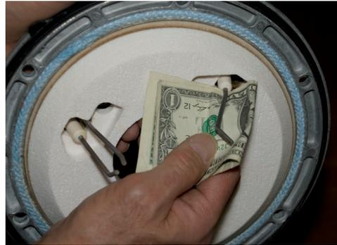
*Fig. B33-1 - Correct way to clean the flame sensor*
