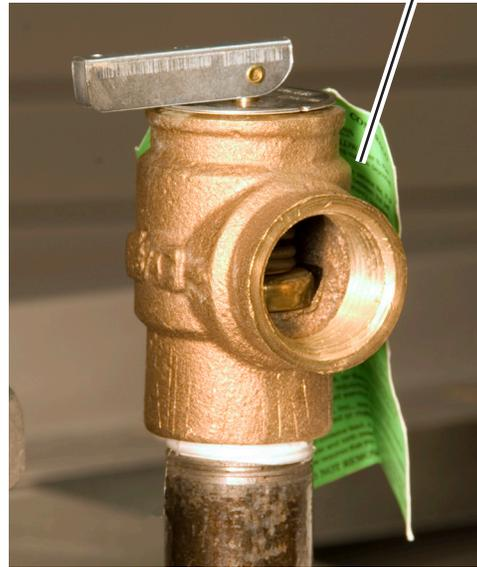
Fig. B31-1 - Pressure relief valve (typical)
