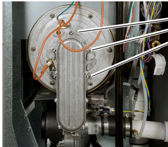
Fig. C5-7 - Removing the front plate with attached air-gas channel and blower
