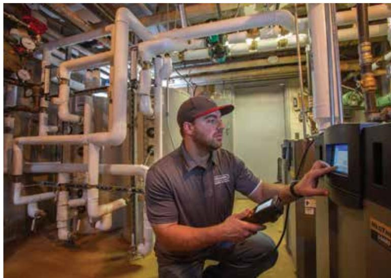
**IMPRESSIVE CONTROLS:** A tech with Denron Plumbing and HVAC LLC checks the controls on a Laars boiler.
