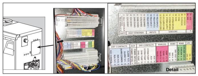
Figure 8. Input and Output Terminal Strips
