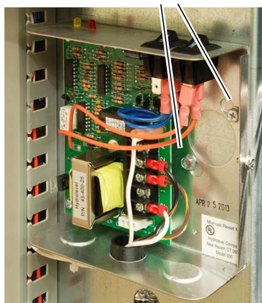
Fig. B6-3 - Control for low water cutoff with cover removed
