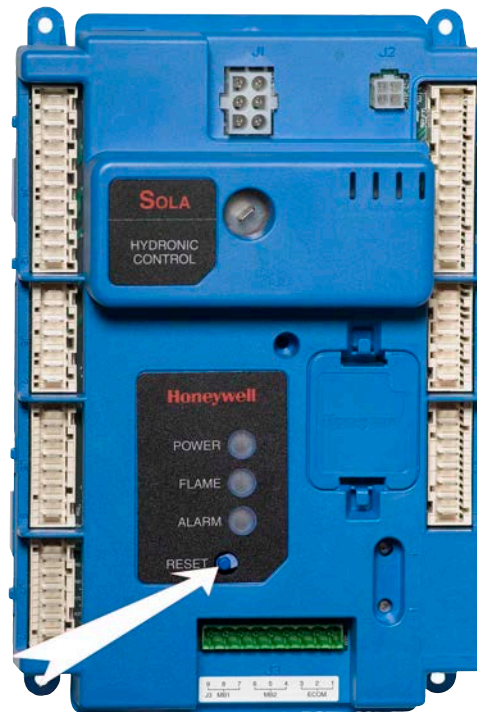
Fig. D6-1 – Resetting the SOLA controller
