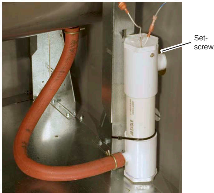
Fig. B17-1 - Small condensate trap assembly (typical)
