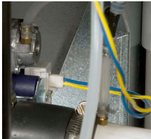
Fig. B11-2 - Wiring connector for gas valve (typical)
