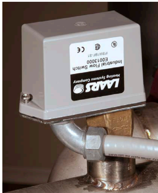
Fig. B9-1 – Typical flow switch installation
