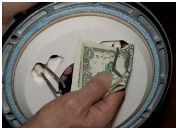
Fig. C5-10 - Correct way to clean the flame sensor
