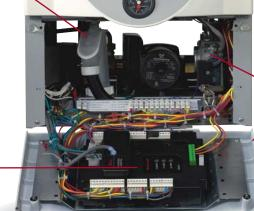
Every Mascot II is equipped with an advanced Laars integrated LCD push button control system, illuminated power switch and pressure gauge. Temperature control, diagnostics, outdoor reset capability and many other functions are seamlessly integrated in this one easy to use center console.
