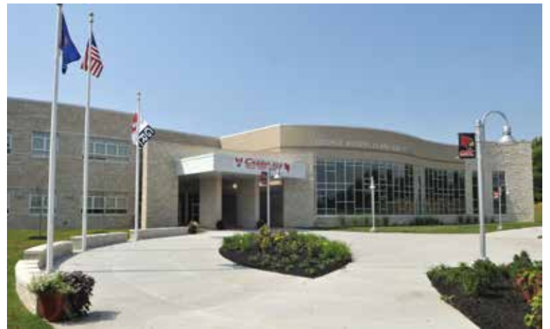
The energy savings are attributed to a 50 percent airflow reduction that chilled beam technology offers versus conventional forced-air distribution methods as well as better humidity control and higher set point temperatures with no trade-off of indoor air comfort.
