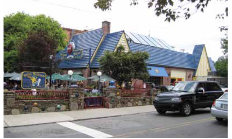
Mellow Mushroom, located in Asheville, North Carolina, installed a solar thermal hot water system as part of its Efficient Heating and Cooling initiative. The system was sized to produce 20 percent of the restaurant’s hot water consumption in a day, and can be expanded to provide more in the future.
