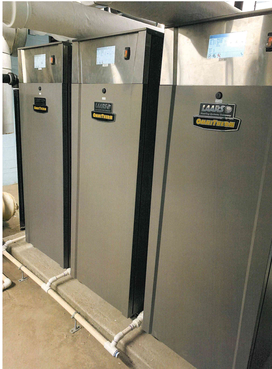
A view of the three new OmniTherm units in the school's mechanical room.
