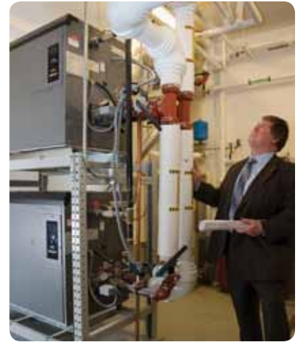
ECI Mechanical Engineer, Don Swick, reviews the boiler installation at Carlos Gilbert Elementary School.
