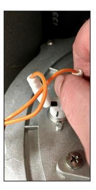
Step 25. Reconnect the gas line to the venturi. Be sure the green paper gasket is seated at each gas line connection. Both the natural gas and LP fuel orifices are tapered. Install the orifice so the taper is facing outward – toward the front door of the boiler. The taper should be visible when installed in the venturi. Tighten both ends of the gas pipe.
