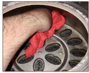
Step 15. If the tube sheet or tubes appear dirty or fouled, flush the heat exchanger. Begin by removing the condensate trap from the flue collector. Remove the four Philips head screws and air hose connected to the blocked condensate switch. Install a short piece of 1" ID hose to the condensate outlet connection on the flue collector. Run the hose to a bucket or drain to catch water while flushing the heat exchanger. Spray water into the fire tubes to flush any deposits through the tubes
