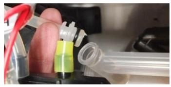
Step 16. Disassemble and clean any debris or build-up from the condensate trap. Ensure the check ball moves freely up and down inside the trap and the clear tube between the condensate trap and air pressure switch is clean and dry. Reassemble and re-install the trap once it is clean and the boiler heat exchanger has been flushed.
