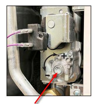
Photo 4. Gas Valve Adjustment Port
